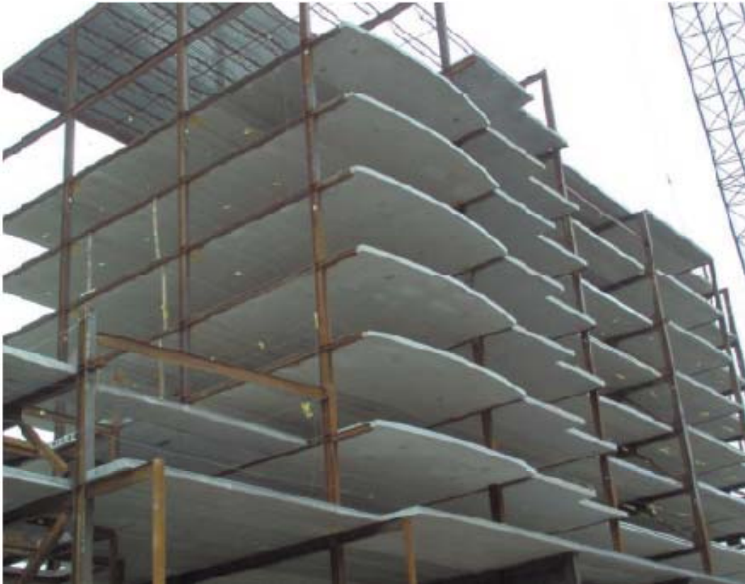
Typical Girder-Slab Structure
